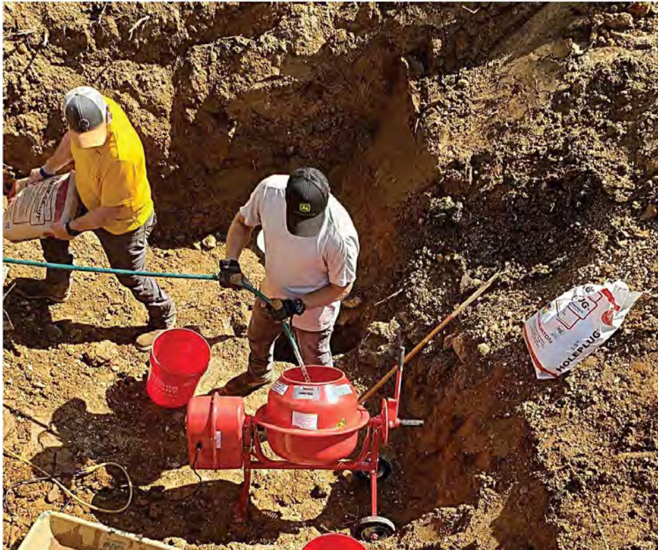
Photograph 8 - Preparing to Abandon bedrock well HR-69Q-MW02 with bentonite Quik Grout.
