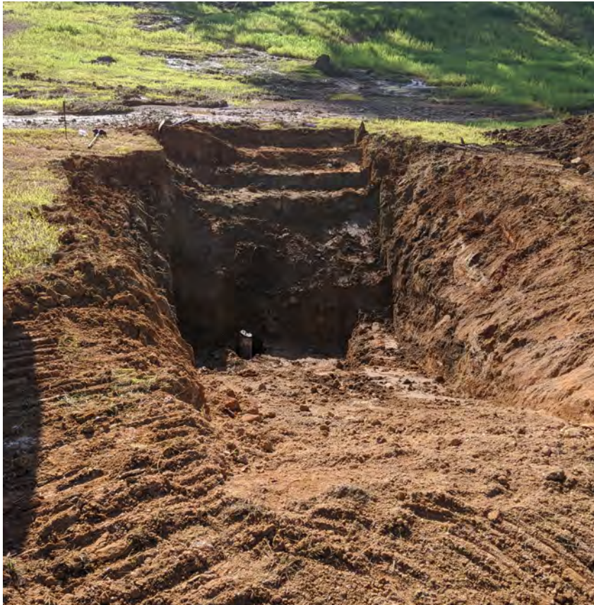
Photograph 6 - Second attempt to abandon HR-69Q-MW02. Outer casing cut off and inner casing cleared at about 9 feet below ground surface.
