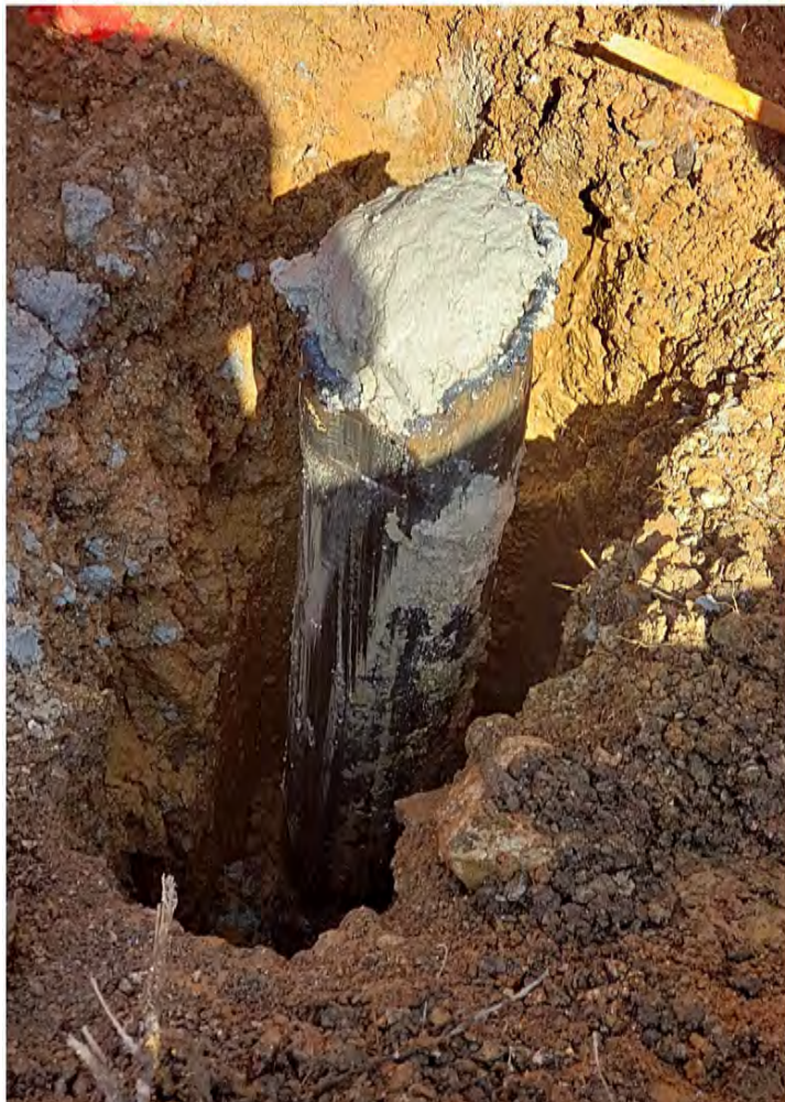
Photograph 10 - Bedrock well HR-69Q-MW02 after sealing with cement/bentonite.
