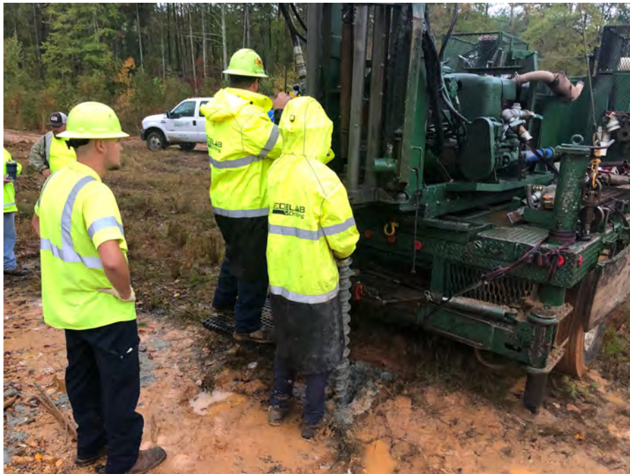
Photograph 2 - Monitoring well HR-69Q-MW01 being over-drilled using hollow stem augers to the full depth of the well to remove well screen and casing
