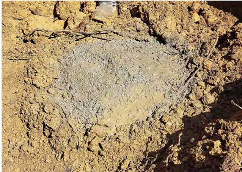
Photograph 11 - Bedrock well HR-69Q-MW02 finished by grouting flush to the ground surface with cement/bentonite.
