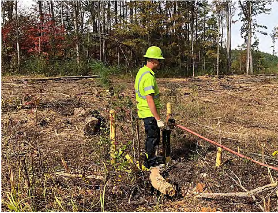
Photograph 1 - Monitoring well HR-69Q-MW01 being grouted in-place from the bottom to top via the positive displacement method (tremie grouting).
