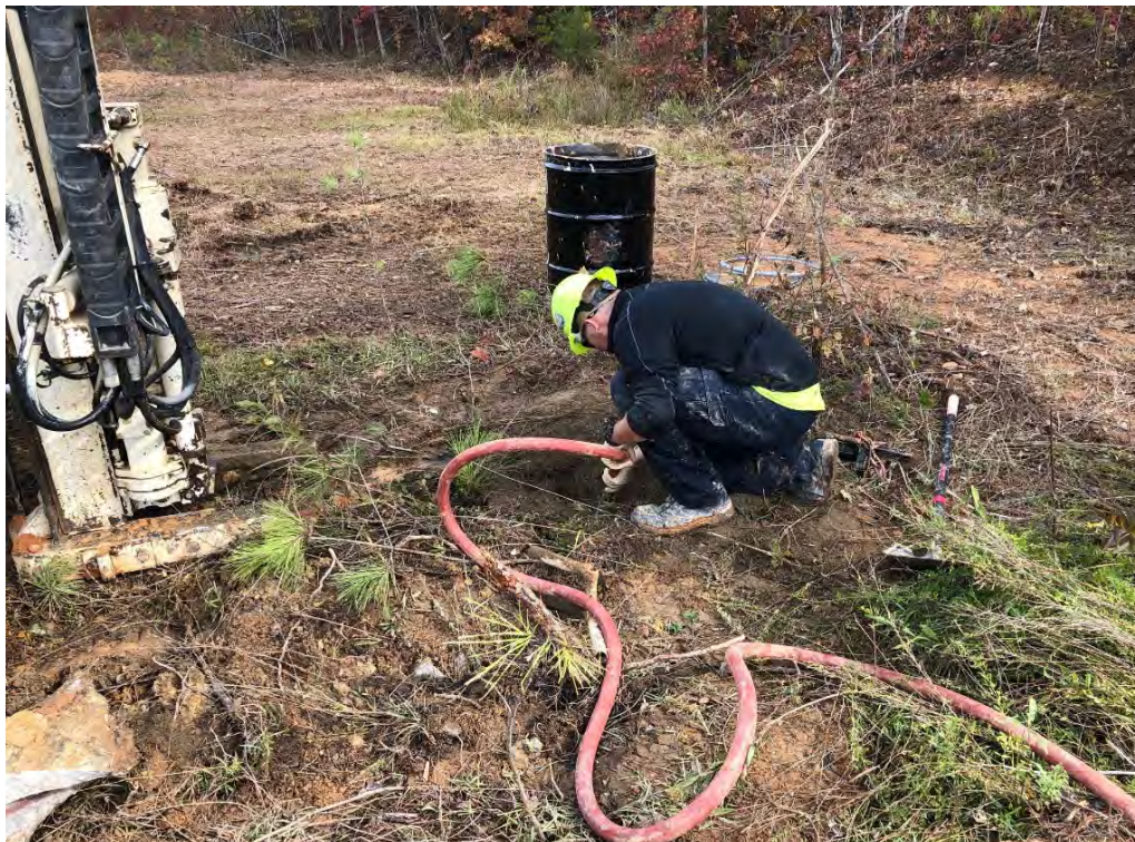
Photograph 3 - View of well being grouted to surface after overdrilling.
