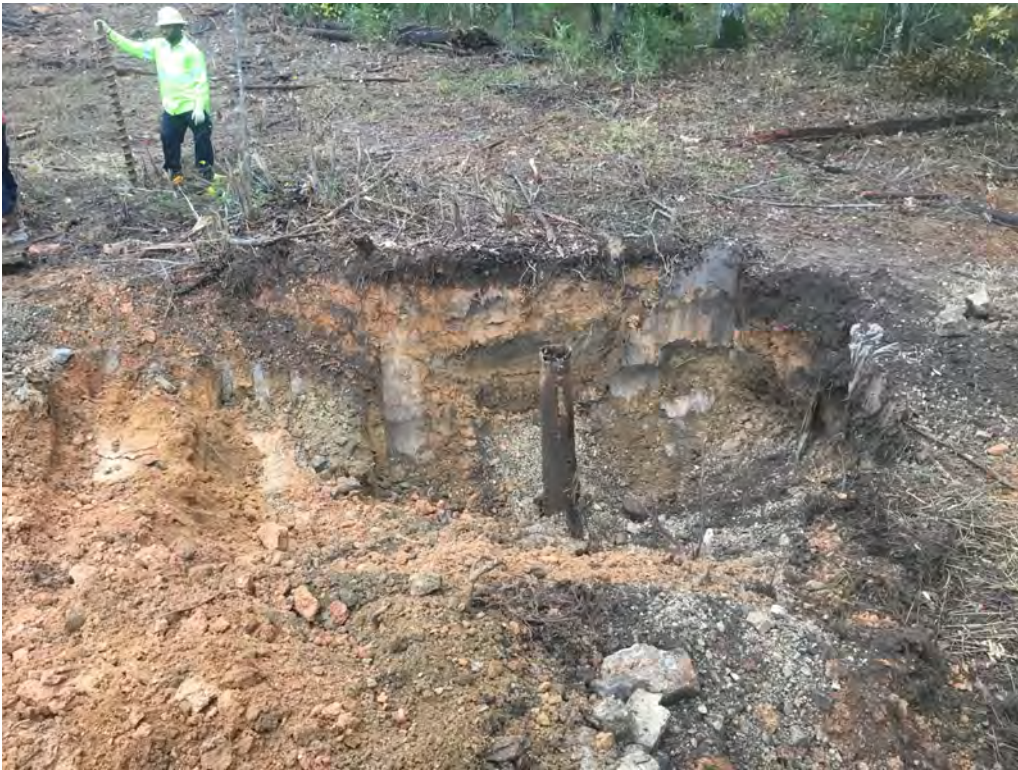
Photograph 5 - First attempt to abandon HR-69Q-MW02. Inner casing plugged to greater than 4.5 feet below ground surface.
