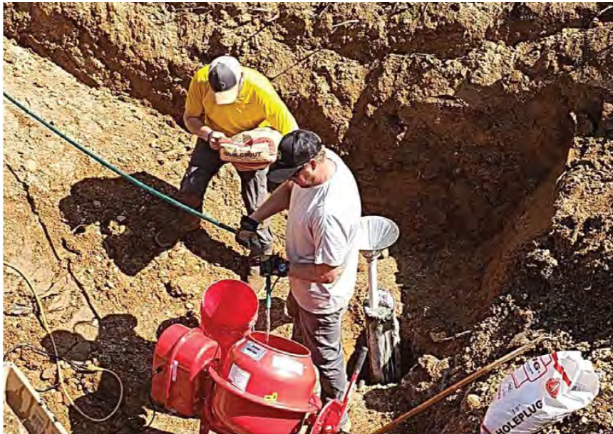
Photograph 9 - Gravity feeding well sealing materials into bedrock well HR-69Q-MW02.
