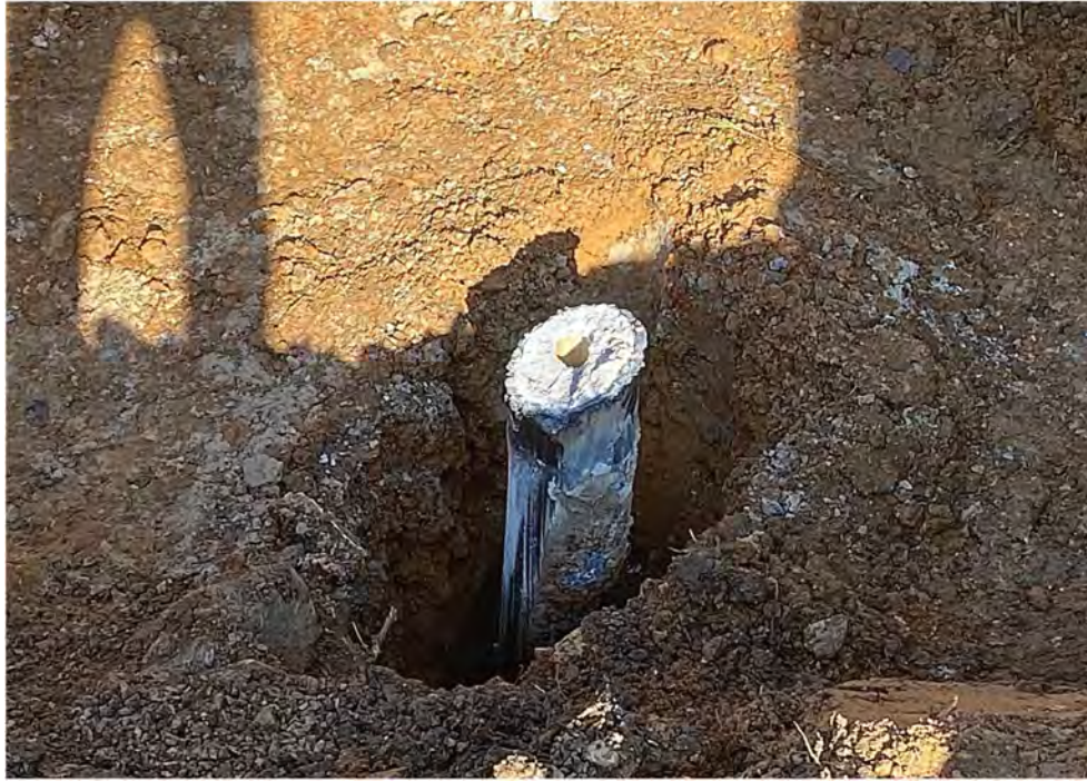
Photograph 7 - Bedrock well HR-69Q-MW02 after excavating, cutting casing, removal of mud and debris manually.
